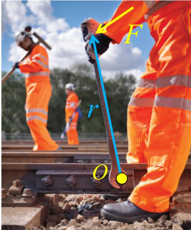
In order to analyze structures subjected to general force systems that can cause rotation, we introduced the concept of the moment of a force about a point
