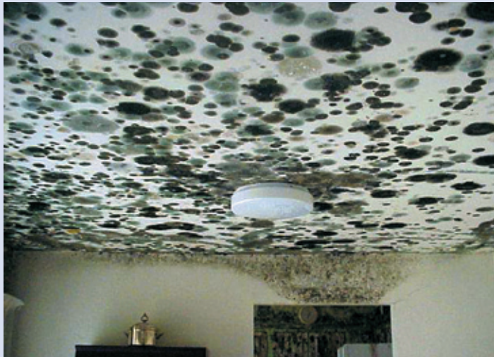
Photo 2: Extensive mold contamination of ceiling and walls
